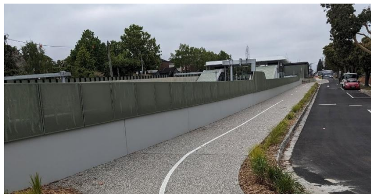
Existing Section of Hawthorn to Box Hill Trail near Union Station
