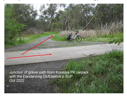
9. The existing informal walking track close to the southern end of the bridge (SUP) because has limited sight lines before/after the bends in the Dandenong Creek/Eastlink path as shown in the photos above.
